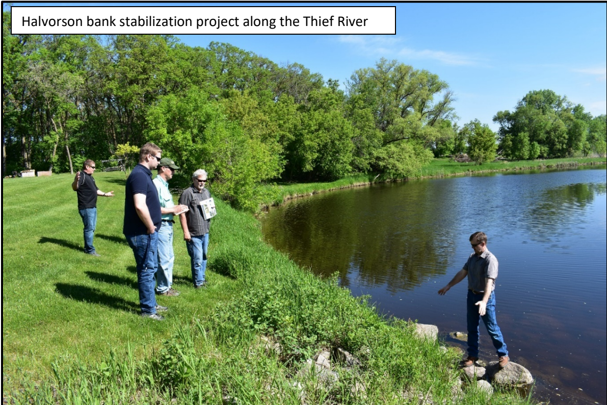
Part of the Halvorson stream bank stabilization project recently collapsed during high flows
